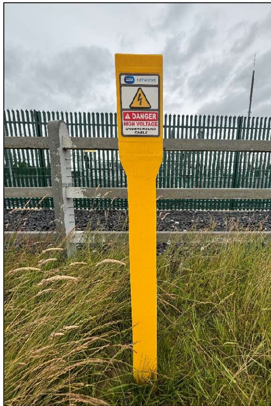
Figure 5-7 Typical Cable Marker Post
